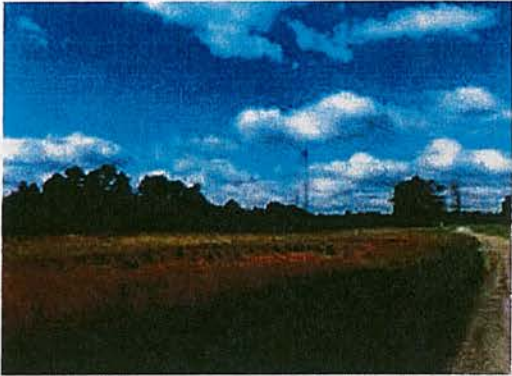
Distant view of cell tower
