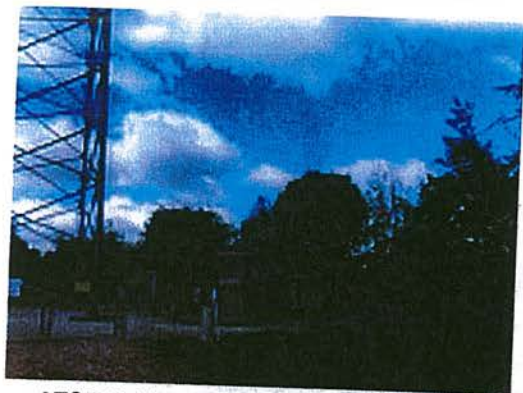
AT&T Utility building under cell tower
