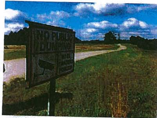
No Public Dumping Sign on Commerce Drive on the east side of subject property
