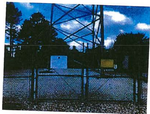
Gate leading to cell tower and utility building
