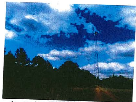
Approaching Cell tower from unnamed road
